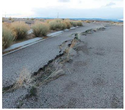
A fissure, or crack in the earth, has displaced asphalt and damaged infrastructure in an uninhabited Enoch subdivision. The fissure is believed to be caused by overdrafting of the underground aquifer, or removing more water than is being recharged each year, according to a Utah Geological Survey study. | Photo by Ashley Langston
