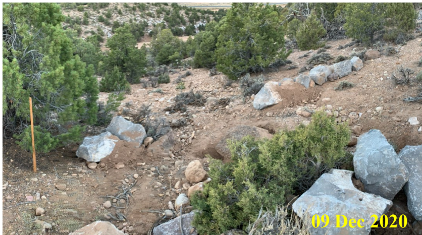
So a Check Dam was started.
