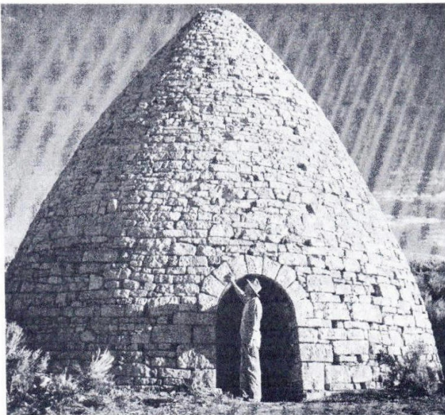
Dr. F. G. Tagert of Austin, Nevada, examines the excellently-wrought masonry of one of the six charcoal kilns at Ward.
