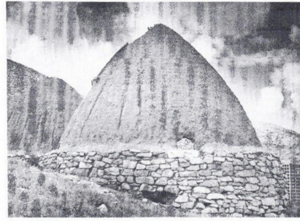
Rock and adobe kiln built at Gold Hill, Utah, 65 years ago.
