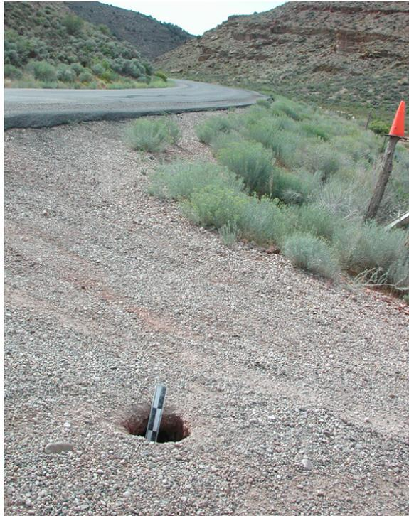
*Figure 7. Evidence for piping below a dirt road, along strike of cracks on the Parowan Gap road (top of photo). Part of scale visible is about 20 cm long (10 cm divisions). View is to the west.*
