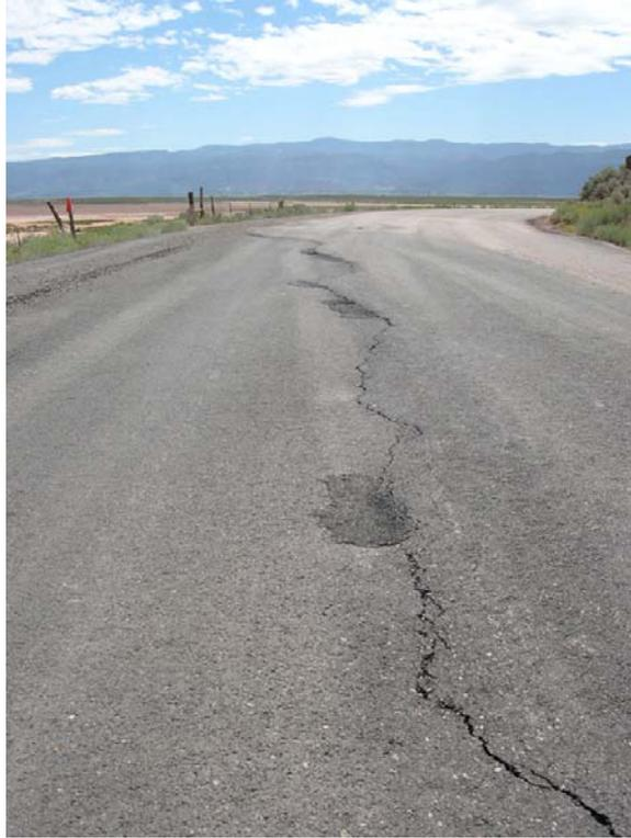
*Figure 6. Hairline cracks along Parowan Gap road. Road patches indicate collapse of subsurface erosional pipes below the surface. View is to the east.*
