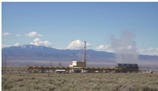
Photo of the Blundell Geothermal Plant
