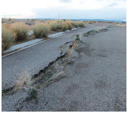
A fissure, or crack in the earth, has displaced asphalt and damaged infrastructure in an uninhabited Enoch subdivision. The fissure is believed to be caused by overdrafting of the underground aquifer, or removing more water than is being recharged each year, according to a Utah Geological Survey study. | Photo by Ashley Langston
